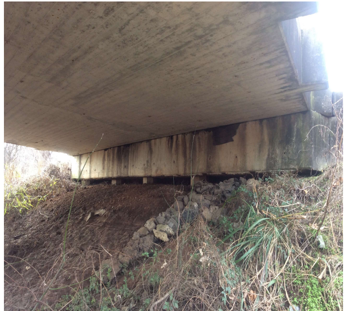
PHOTO 2 Description End slope - Bent 1 (settlement)
