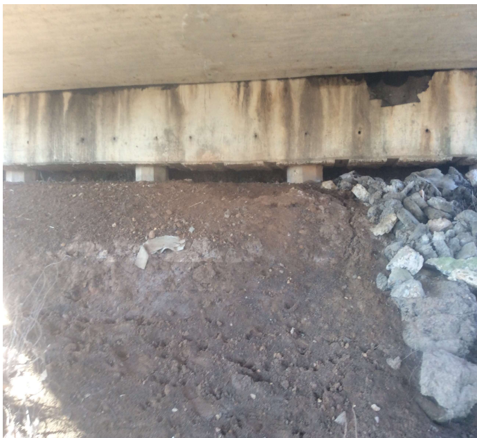
PHOTO 3 Description Erosion at bent 1 abutment under cap has exposed piles .
