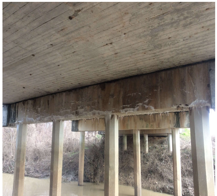
PHOTO 2 Description Cap - Bent 3 (efflorescence)
