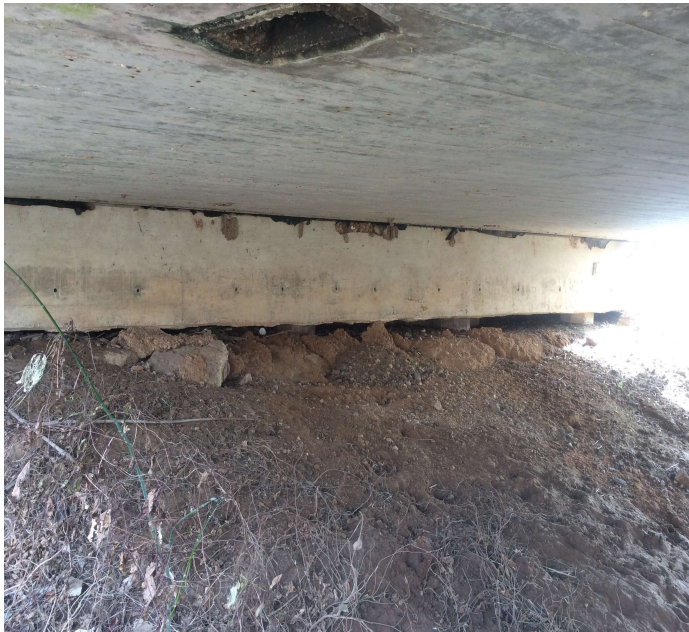
PHOTO 1 Description End slope- Bent 6 (settlement)
