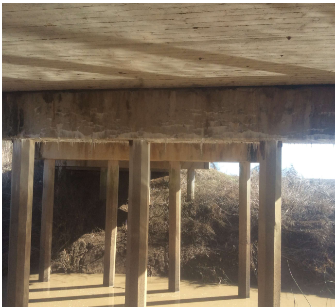
PHOTO 3 Description Bent 3 cap has very excessive amounts of cracks with efflorescence the length of cap .
