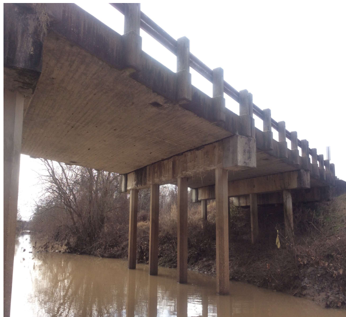
PHOTO 1 Description Cap - Bent 3 (efflorescence & patches)
